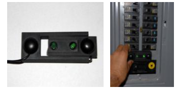
Figure 3: Easy-to-install power meter that a user can stick-on to the outside of a breaker panel.
